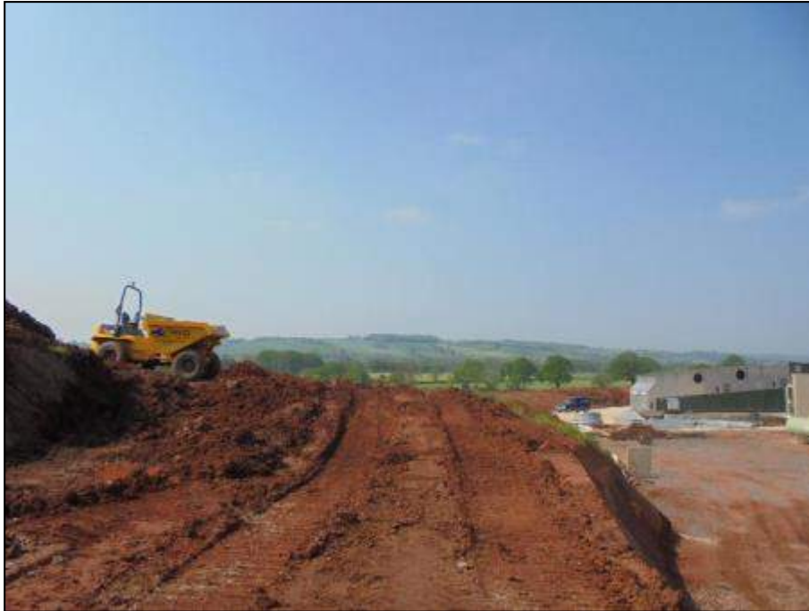
Photo 3-2 The area of bund terraced into the slope on the north-eastern boundary of the application site. Taken from the north-east of the site looking south
